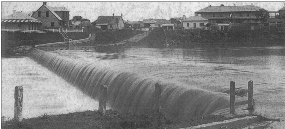
Figure 25: Undated photograph (c. 1890-95) looking south over the Marsden Street weir. The rebuilt 'Riverside' is visible on the left, while the 'Niagara' is the large building behind it (from AHMS 2011:128)
