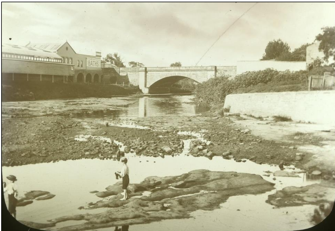
Figure 21: View of Lennox Bridge from the west (c.1900). The study area is on the right. ( http://handle.slv.vic.gov.au/10381/46231 )
