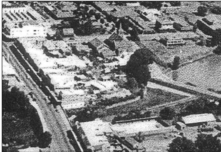
Figure 31: 1938 oblique aerial photograph looking south over the subject site. (AHMS 2011:142)
