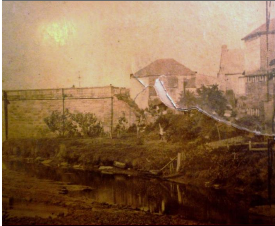
Figure 20: Detail of an undated view of Lennox Bridge from the west. To the right of the bridge are the buildings occupying the eastern side of Allotment 1A (Items 7, 10 and 48). At the extreme right is a three storey building of unknown function (Item 47) (from AHMS 2011:119)
